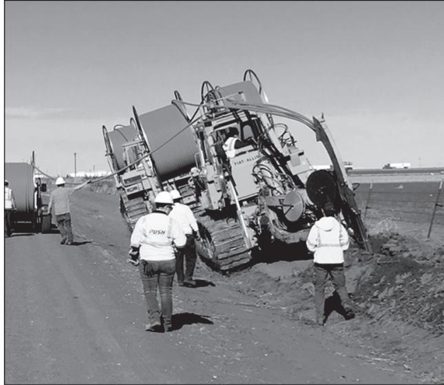
**WTRT/WTS contracted workers with Push Inc. of Rice Lake, Wisconsin plow in duct that will have fiber-optic cable injected into it near Bushland. The project will ultimately see six miles of fiber installed to feed new housing developments in the Bushland area. It's part of efforts to better service customers with fiber to the premise. Once fiber is injected connections will be spliced.**
